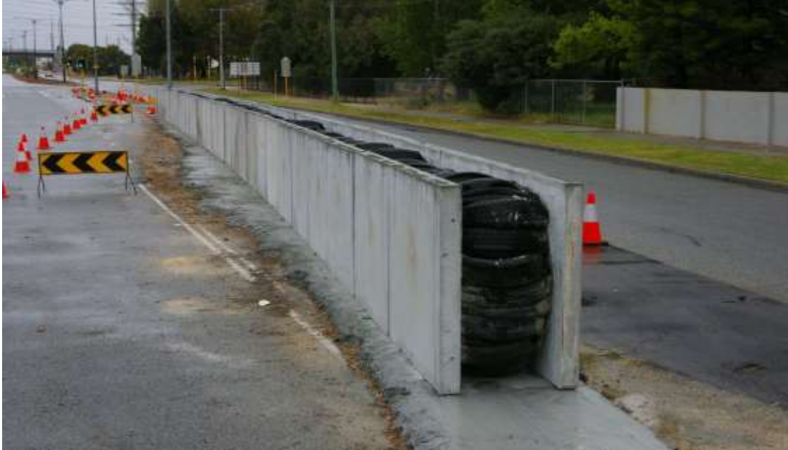
Figure 12: Innovative use of used tyres and recycled concrete in a retaining wall
